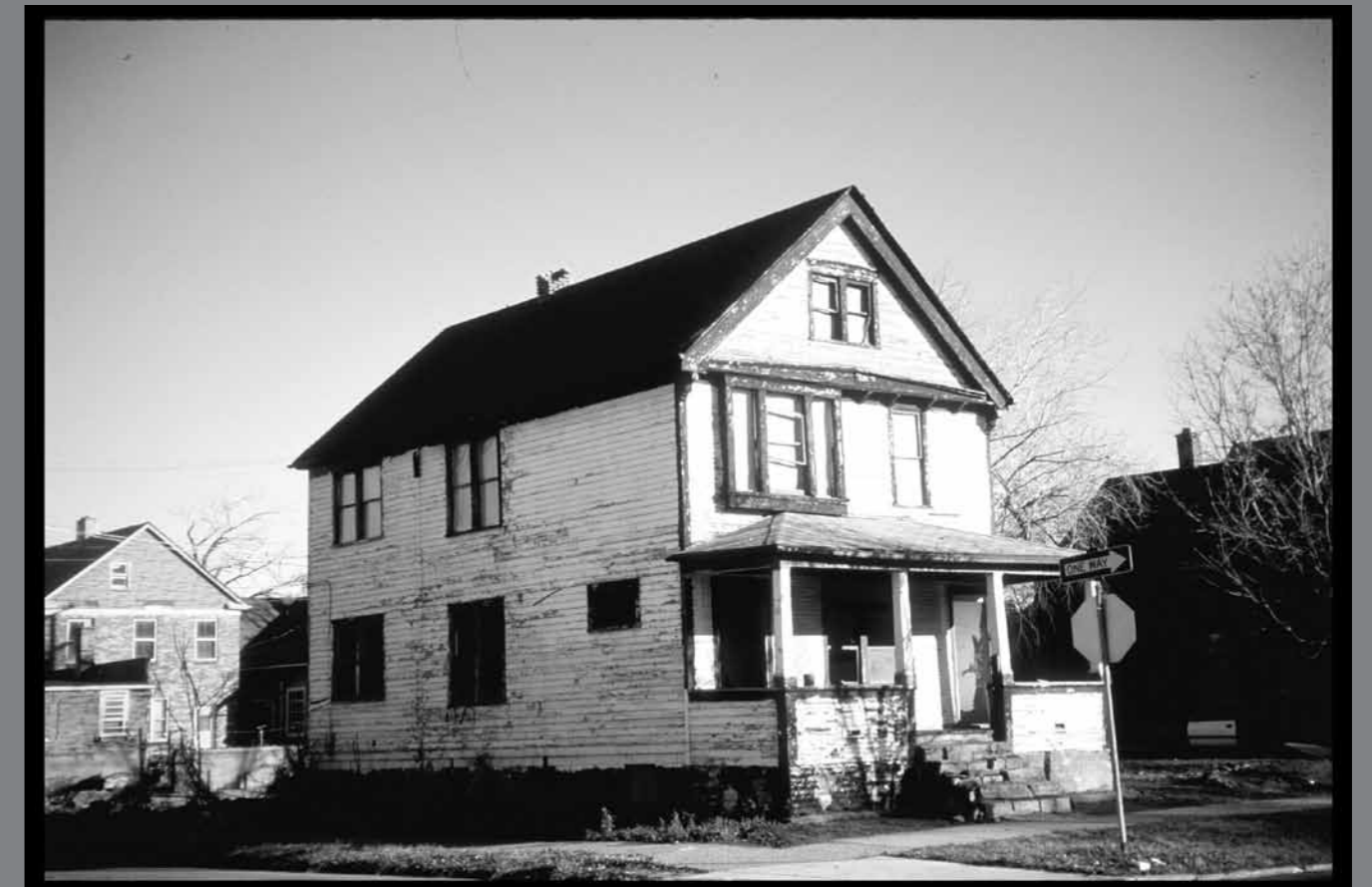
The Detroit House – North West View Designer/photographer: Jonsara Ruth, 1998
